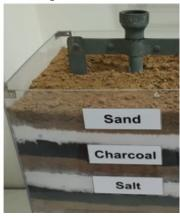
The installation of salt-charcoal type earthing is not done properly. They just mix up and fill up the pit. Even they use lesser depth of pit and mixture.
